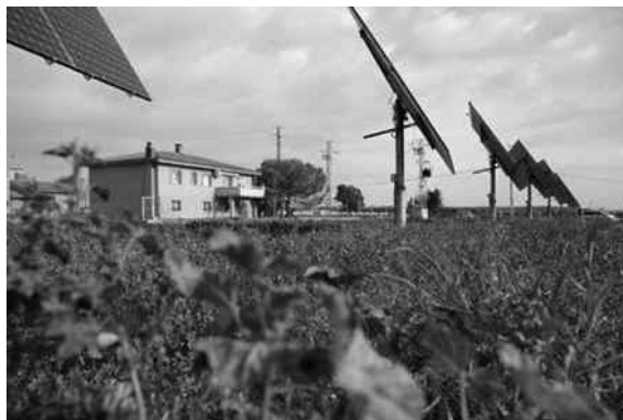
FIGURE 15.7 Solar installations in Germany. (SMA Solar Technology AG.)
