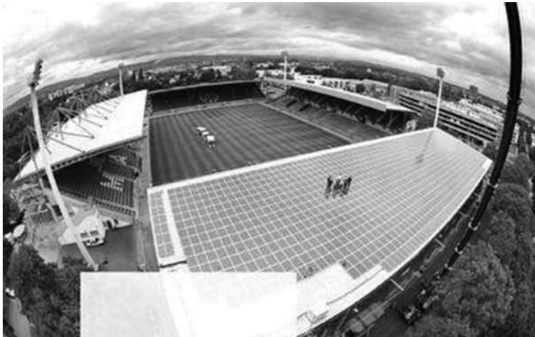
FIGURE 13.21 Solar applications in a sports stadium in the city of Mainz in the state of Rheinland-Pfalz in Germany. (SMA Solar Technology AG.)
