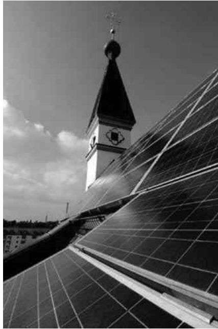
FIGURE 15.8 Solar applications on the roof of Munich Temple in Germany. (SMA Solar Technology AG.)
