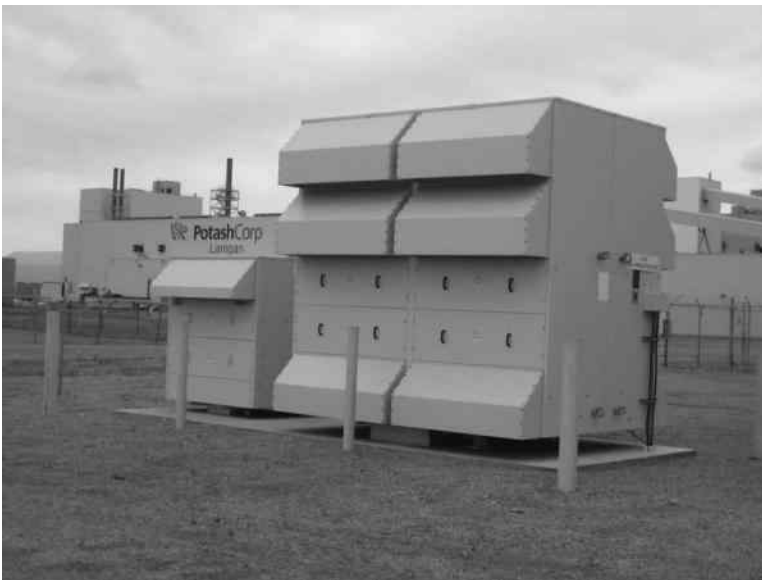
FIGURE 3.5 Outdoor three-phase dry-type resinbloc transformer. (Courtesy of ABB.)
