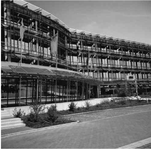
FIGURE 13.20 Solar applications on a building in the city of Laatzen in the state of Niedersachsen, Germany. (SMA Solar Technology AG.)
