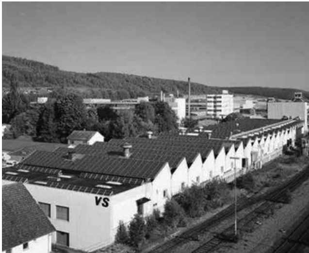
FIGURE 13.23 Solar rooftop applications in the state of Baden-Württemberg, Germany. (SMA Solar Technology AG.)
