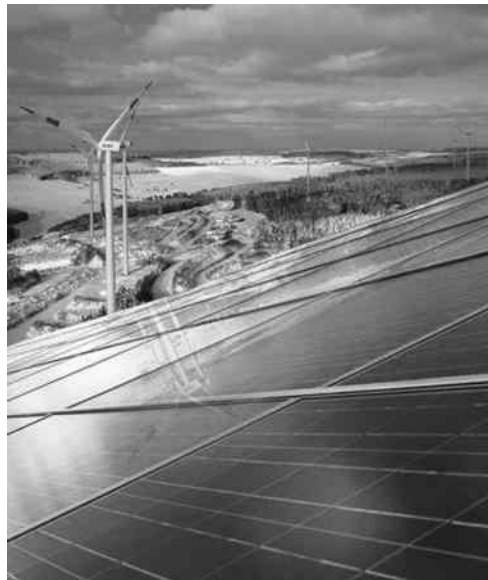
FIGURE 15.6 Solar and wind turbine applications in the state of Rheinland-Pfalz in Germany. (SMA Solar Technology AG.)
