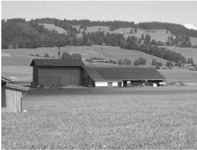
FIGURE 13.17 Solar applications on the rooftop of a barn in Bayern, Germany. (SMA Solar Technology AG.)
